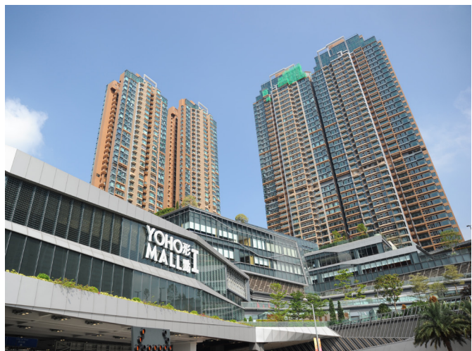
Figure 12: Large-scale shopping mall in Yuen Long, YOHO MALL
