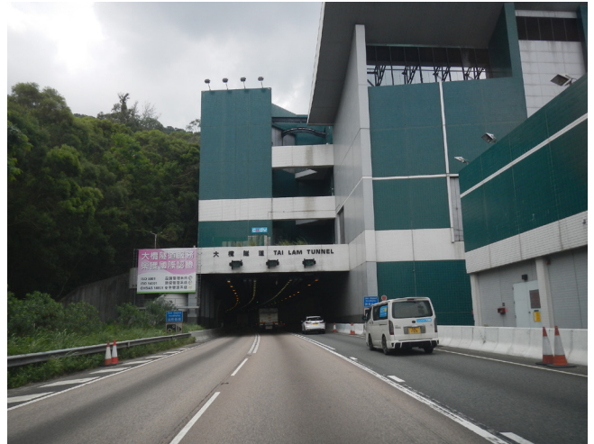
Figure 23: Tai Lam Tunnel
