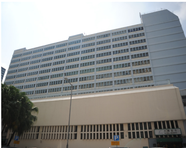
Figure 16: Yuen Long Government Offices
