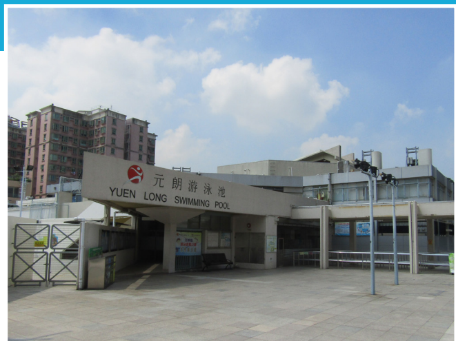
Figure 20: Yuen Long Swimming Pool
