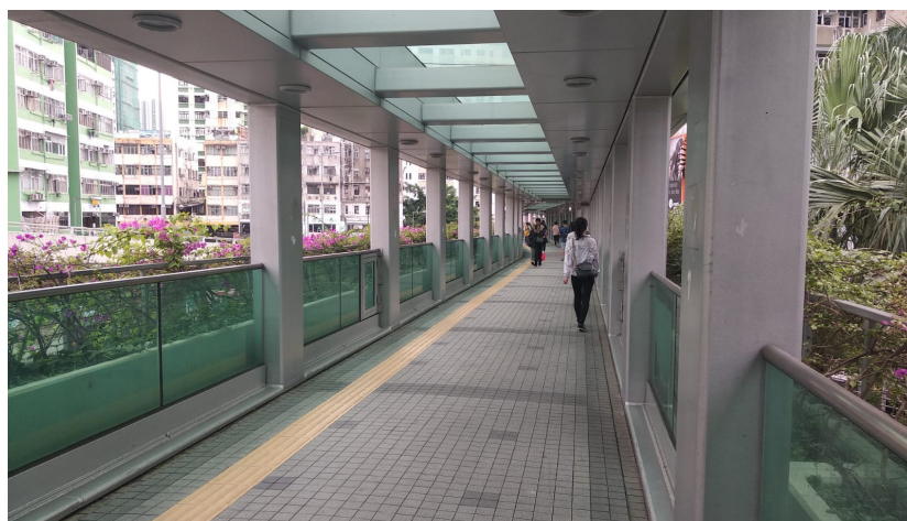
Figure 40: Pedestrian footbridge in Tsuen Wan
