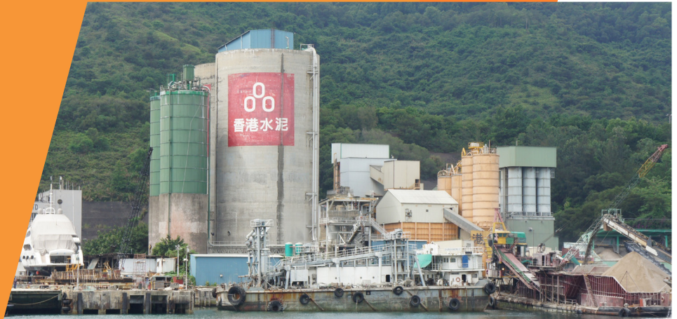
Figure 17: Concrete batching plants in Tsing Yi
