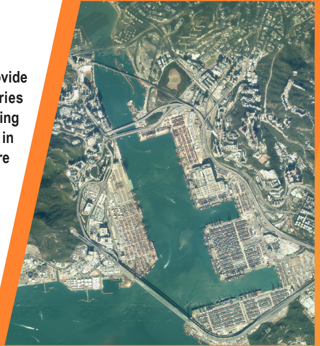
Figure 14: Container terminals on both sides of Rambler Channel
