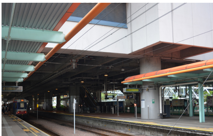
Figure 25: TSW Light Rail Transit Station
