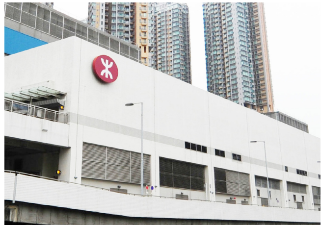
Figure 4: Tuen Ma Line Tuen Mun Station
