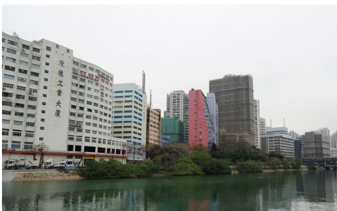
Figure 28: Flatted factories to the West of Tuen Mun River Channel
