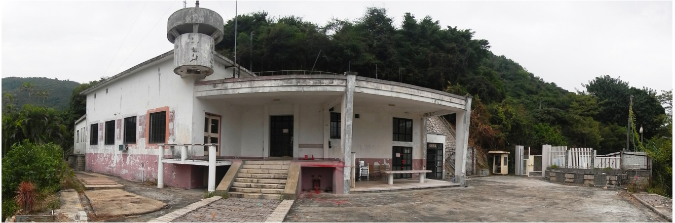
Figure 20: Ex-Tiu Keng Leng Police Station
