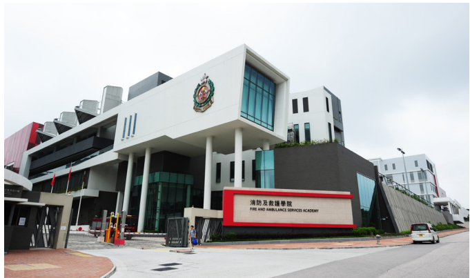
Figure 15: The Fire and Ambulance Services Academy
