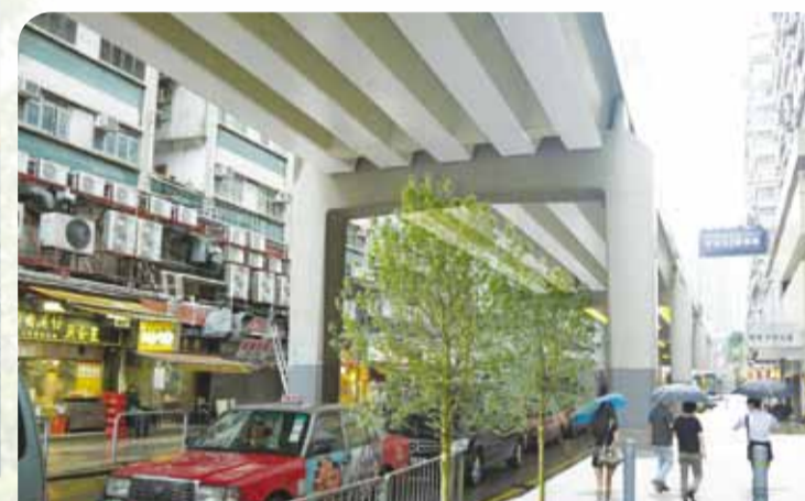
優化後的民裕街街道環境(模擬圖) Streetscape of Man Yue Street after enhancement (Photomontage)
