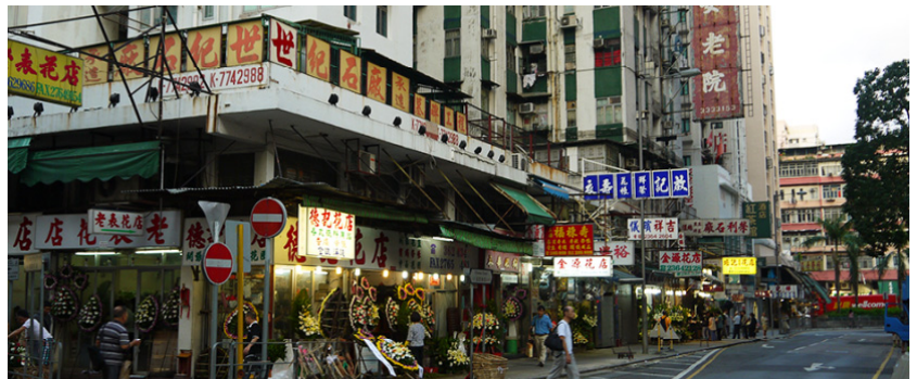
Existing condition of Wuhu Street, Winslow Street, Gillies Avenue South Area, Hung Hom
