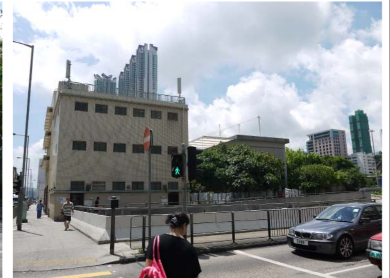
4 Pedestrian walkway adjacent to Kai Tak Tunnel Entrance is segregated by Kowloon City Road.
