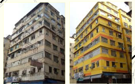
1&3 Shim Luen Street Before and After Rehabilitation
