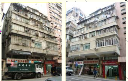
41-45 Pau Chung Street Before and After Rehabilitation
