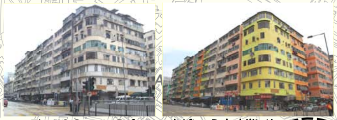
The 13 Streets Before and After Rehabilitation
