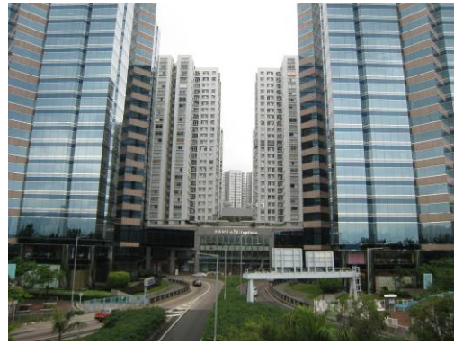
P14 Gap between Cityplaza Three and Four facing immediately the podium of Phase 2
