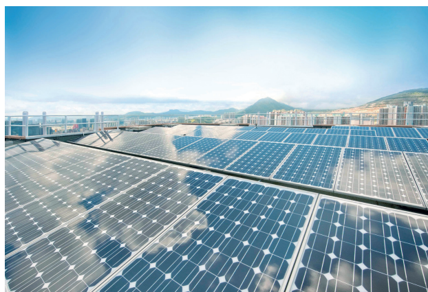
藍田邨天台上的太陽能光伏板 Electric Solar panels installed on roofs of Lam Tin Estate
