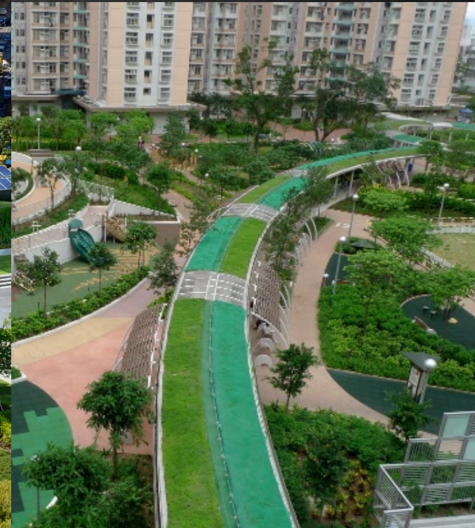
Green Covered Walkway at Sau Mau Ping South Estate
