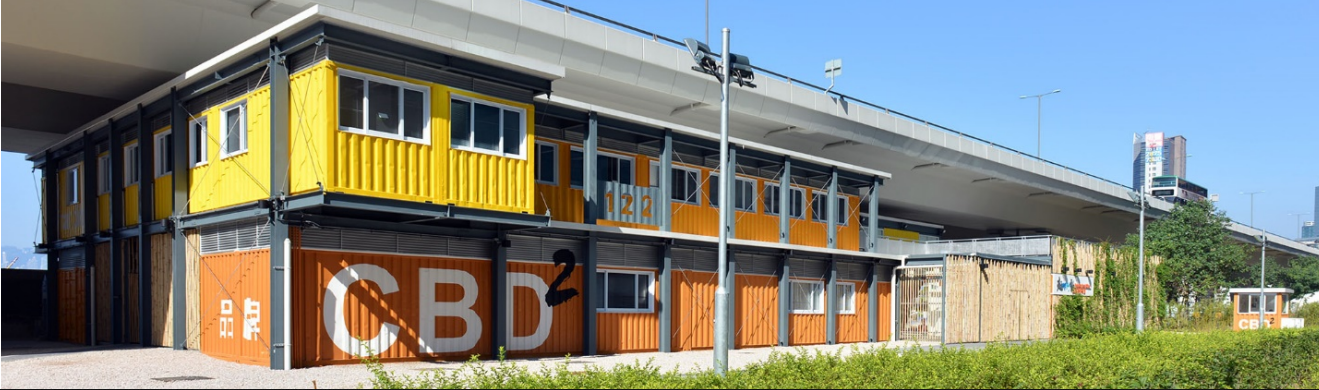
Energising Kowloon East Office built from recycled containers
