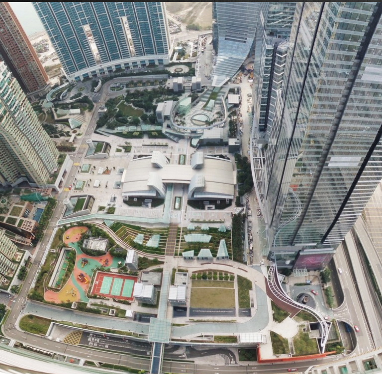
Kowloon Station / Elements Mall shared podium garden
