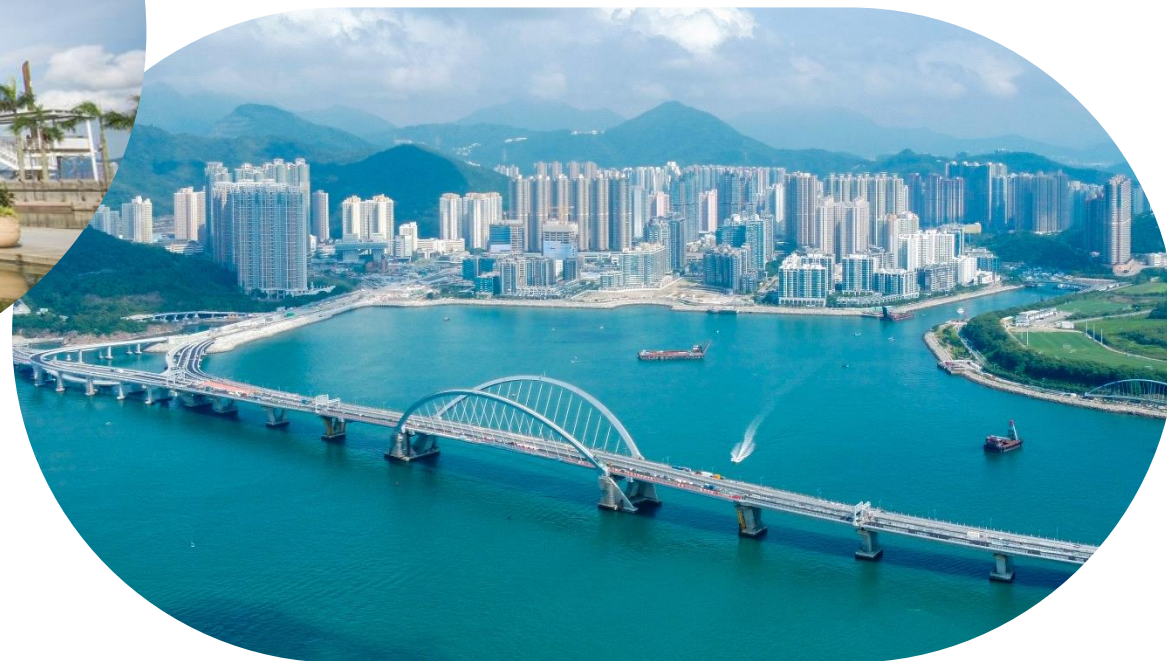
Tseung Kwan O Cross Bay Bridge
